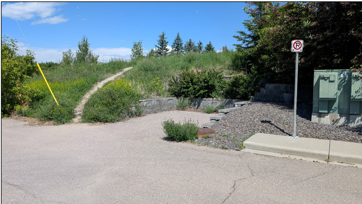
Existing Turnaround at West Terminus of Erlton Terrace SW
